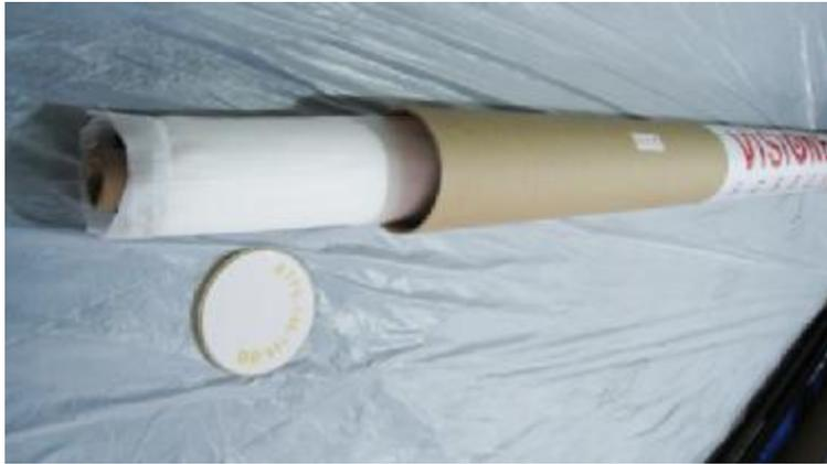
Open the screen fabric (A4) packaging, and place the black backing fabric to one side for the moment. With gloves on, flatten and spread out the screen fabric (A4) over the frame.
