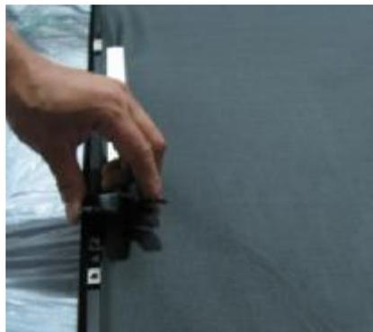
3. Place M6 hex screws (P7) into the mounting hole, and connect it with the square nut in the frame's groove. Fasten the screw with the hex wrench and fix the wall-mount in place.
